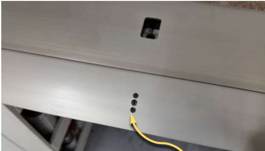
Image showing additional holes to inject spabond.
